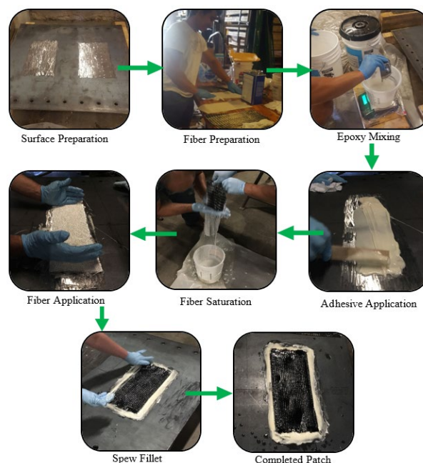
Figure 5: FRP patch retrofit application process
